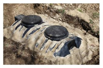
NFPA 30 and 31 address requirements including type and location of tanks. This includes distance to buildings and property lines, and protection against movement/upheaval caused by flooding or increased groundwater levels. (www. nfpa.org)
